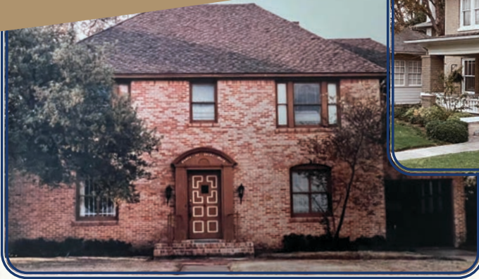
Braeswood Home Office
